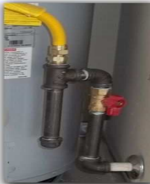
Samples of correct sediment trap installations
